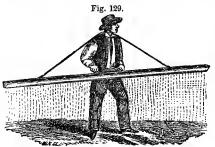
A very simple machine for sowing grass, as well as other small seed, by hand, is shown in the annexed figure. It consists of a light trough, containing the seed, which is distributed through holes in the zinc bottom by the vibrations of a notched rod, and any desired quantity of seed accurately regulated.
