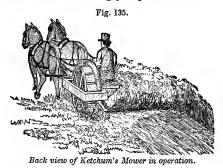
represents Ketchum's mower in operation as seen from behind, cutting an even swath five feet wide as fast as the horses advance.
