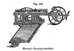
As the straw collects on this platform, it is raked off in successive bunches for binding by a man who rides on the machine for this purpose.
